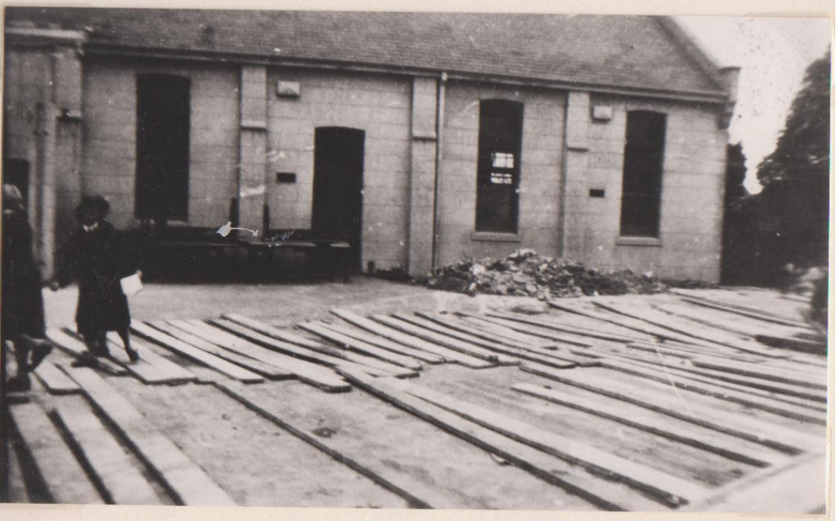
Eymard Temby Hall freestanding prior to 1950 – use your imagination – now the West Wing
